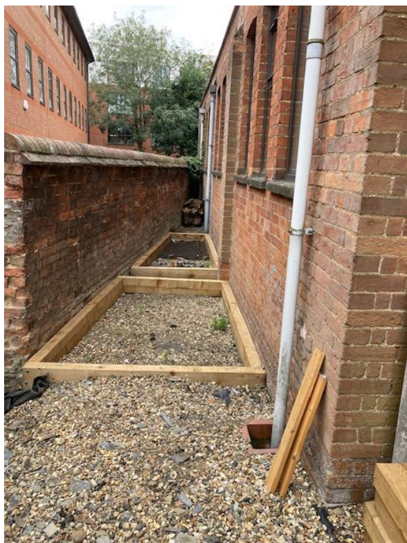
It's a frame up! Our first two bed frames for phase 1.
