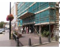
A £15,000 scheme is underway during August to ensure the masonry at the front of the church remains safe. Some pieces fell off last summer and whilst a survey showed no immediate danger, contractors are examining each piece of stone and adding metal pins as well as mortar to ensure it remains firmly in place. Kevin Hardern, the Resources Coordinator explained, "The contractors are used to working with churches and aim to be finished for Helen's welcome service."
