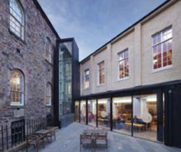
Left: Making connections – church building and Epworth Halls joined
