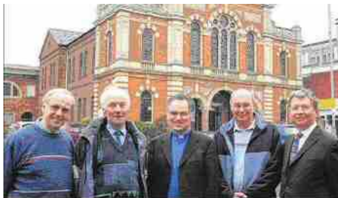
Some members of the Steering Group in front of the church with its off street entrance to the coffee bar. The entrance to the Community Centre and redevelopment area is at the back to the left. Photo: Courtesy The Bucks Herald .
