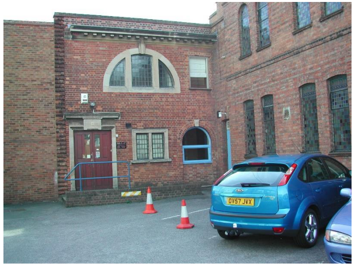
The community centre back entrance ten years ago.
