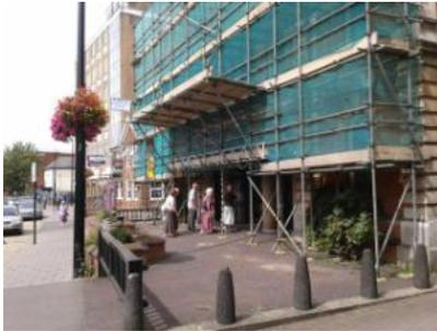
**A £15,000 scheme** is underway during August to ensure the masonry at the front of the church remains safe. Some pieces fell off last summer and whilst a survey showed no immediate danger, contractors are examining each piece of stone and adding metal pins as well as mortar to ensure it remains firmly in place. Kevin Hardern, the Resources Co-ordinator explained, "The contractors are used to working with churches and aim to be finished for Helen's welcome service."
